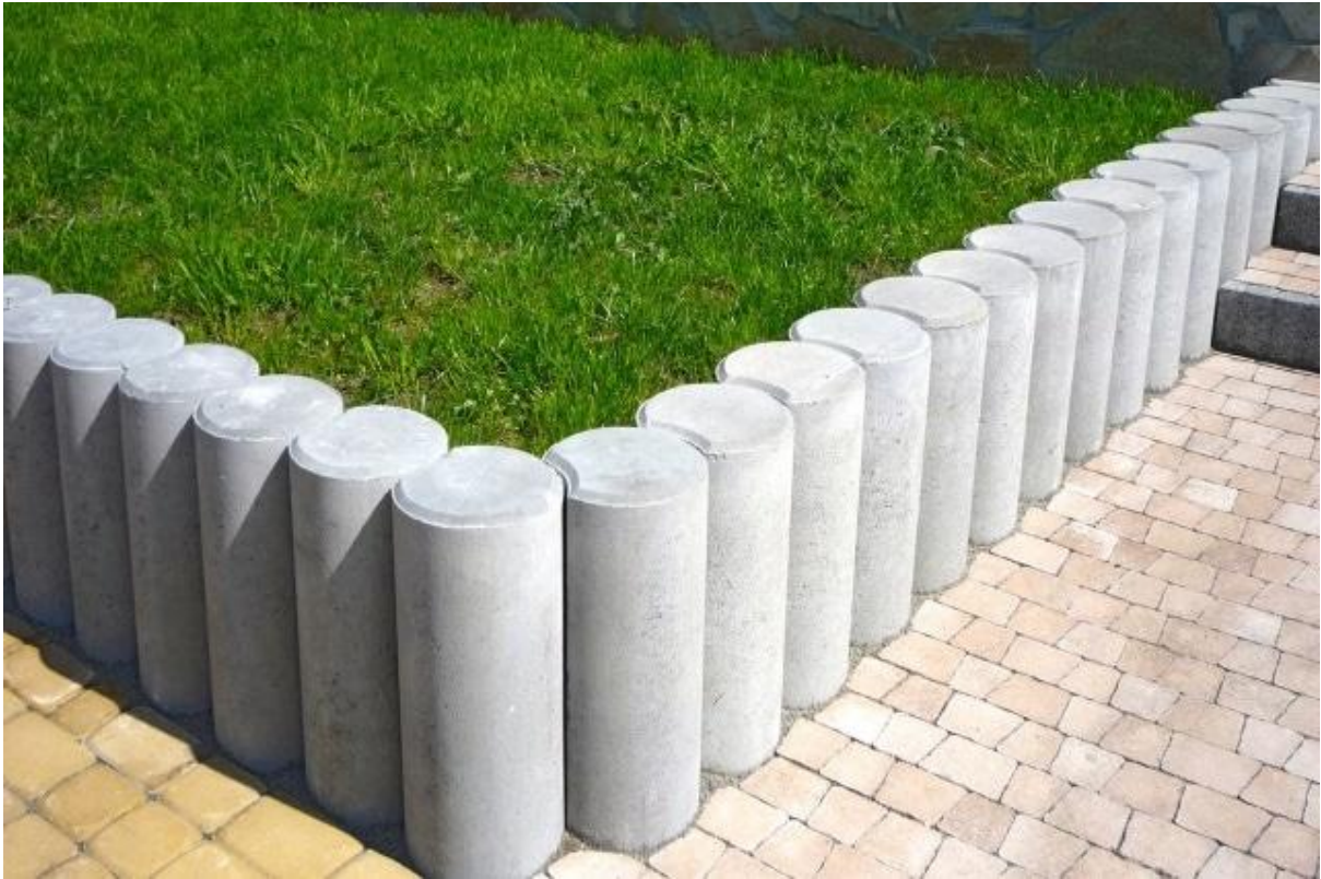
Very durable garden edging make by using PVC downpipe as mold
